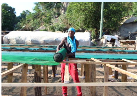
Installing innovative drying rack
